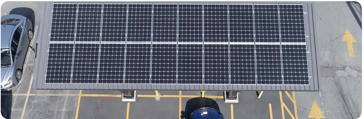
Charging stations, such as this one in Legends Parking Lot, provide infrastructure for an ever-expanding fleet of electric vehicles on campus. Currently, there are five EV charging stations on campus, four of which are solar powered (grid tied).
