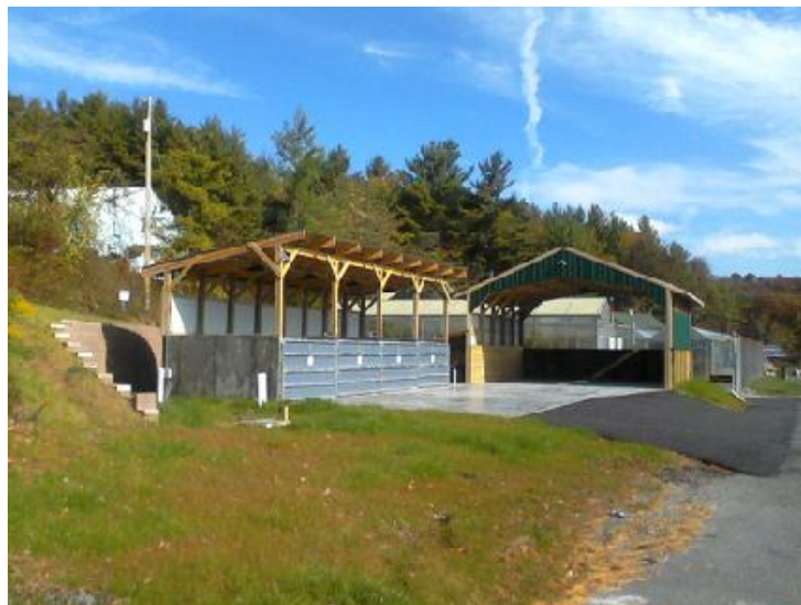
Figure 7: Newly constructed compost facility next to biology greenhouse off of State Farm Rd.
