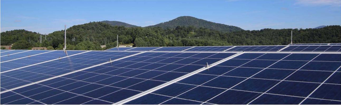
The PV system on the roof of Leon Levine Hall is comprised of 214 panels, with 57.8kW of capacity.
